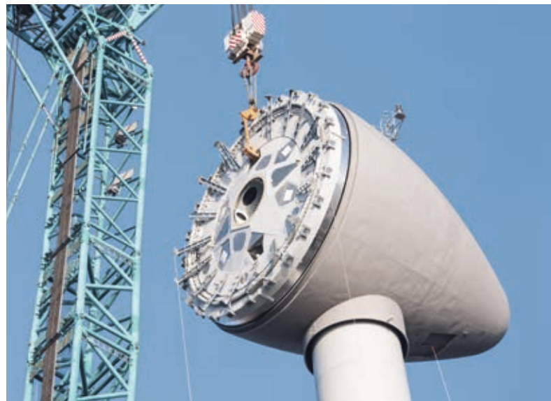
Foto: Installing rotor house at the top of a new Dutch wind turbine © Kruwt, fotolia.com
